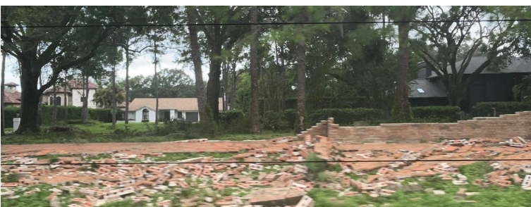
Hurricane Milton Damage
